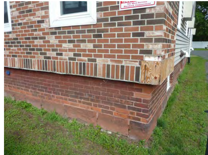
Cleaning and repairs to brick are shown periodically over the plan. Note exposed original stone and brick foundation at southwest corner of building.
