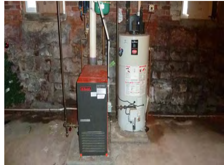
Gas-fired boiler is shown to be replaced mid-plan and the domestic hot water heater early and late. Note signs of historic water infiltration on wall behind.
