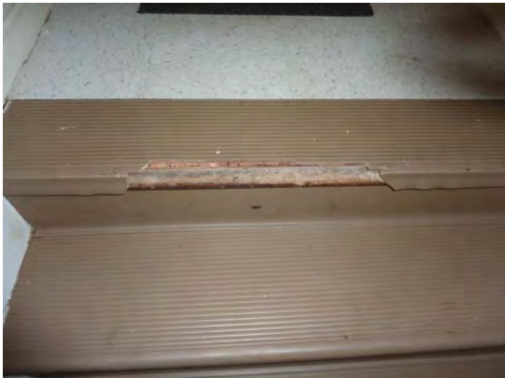
Typical worn or damaged rubber stair tread/riser and vinyl flooring is shown to be replaced early and late in the plan base on EUL and condition.
