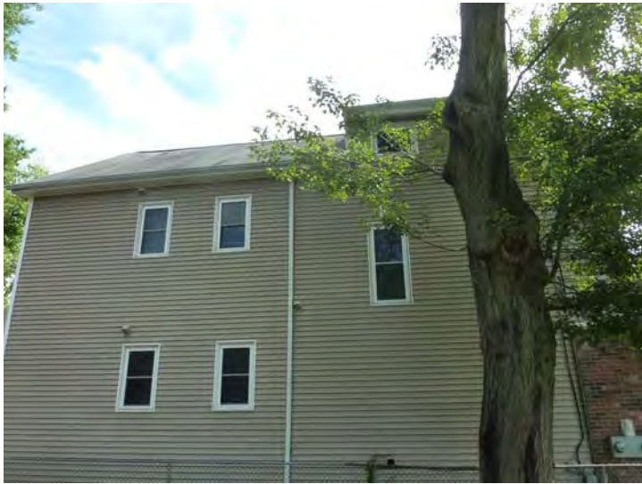
Windows, vinyl siding and roofing are all in good condition and shown to be replaced mid-plan based on EUL and condition.
